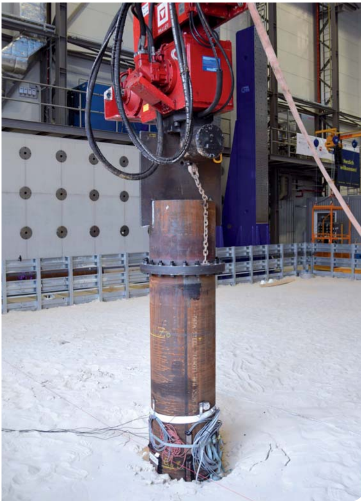
Seabed in the model layout: Construction methods, such as the gentle vibrating in of steel piles, are examined in the test center. © Fraunhofer IWES
