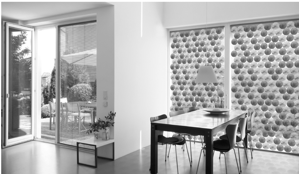
The façade element operates using integrated shape-memory alloys and so doesn't require an external power source. (© Wilm Ihlenfeld/Fotolia, Fraunhofer IWU) | Picture in color and printing quality: www.fraunhofer.de/press
