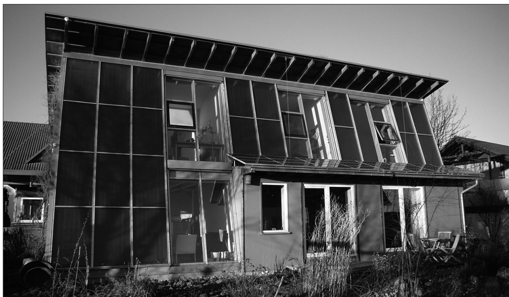
Solar-Active-Houses get most of their heat from the sun. Researchers carried out scientific tests to explore how this energy concept can be optimized further. (© Klaus Lambrecht, solaroffice.de) | Picture in color and printing quality: www.fraunhofer.de/press
