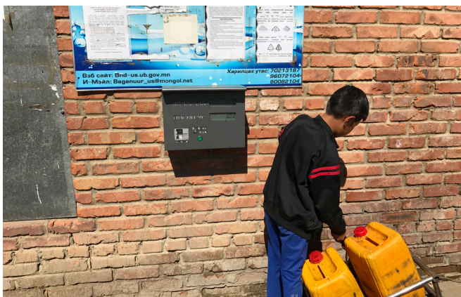
Automatic payment at a water kiosk © Fraunhofer IOSB-AST | Picture in color and printing quality: www.fraunhofer.de/en/press
