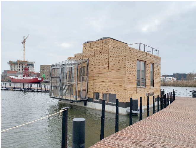
Picture 1: One of the first houses to be anchored.
