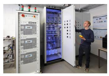
Picture 3: Work on the main distribution neutral unit for the DC test grid at Fraunhofer IISB.
