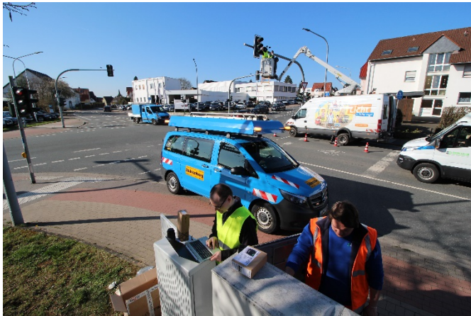
Picture 1 The “KI4LSA” project aims to provide smart, predictive traffic light changing using artificial intelligence. High-resolution cameras and radar sensors gather detailed traffic information.
