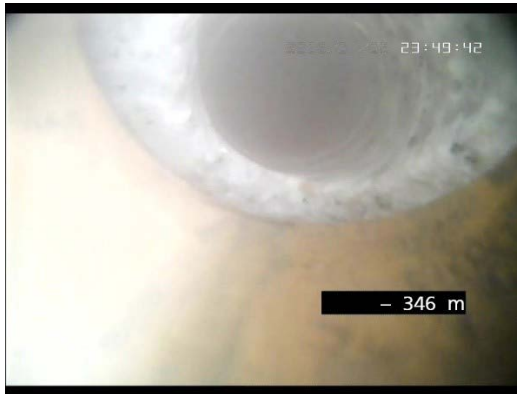
Fig. 3 View of a freshly drilled side arm at 346 meters. The micro drilling turbine milled out the granite rock cleanly.
