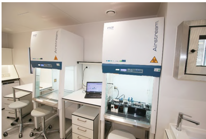
Fig. 2 Two modular class II safety workbenches for BSL-2 work
