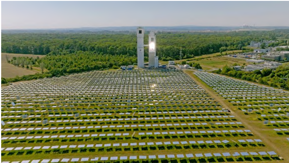
Fig. 1 Aerial view of the solar tower and mirror field of DLR, Jülich. The mirror field concentrates the solar radiation onto the solar tower and heats up the solar receiver.
