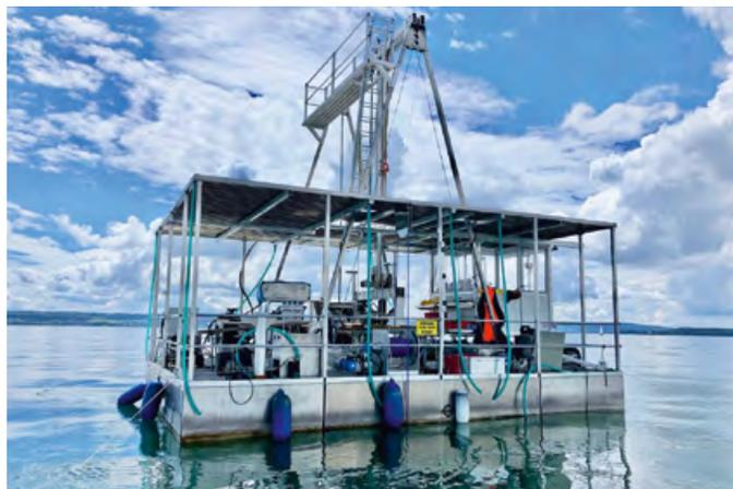
The hammer drill is operated from a compact floating platform.
