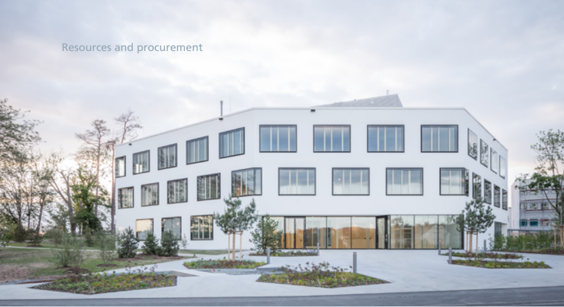
The newly constructed gold-certified building at Fraunhofer IWKS in Alzenau Photo: Rainer Taepper/ Fraunhofer IWKS
