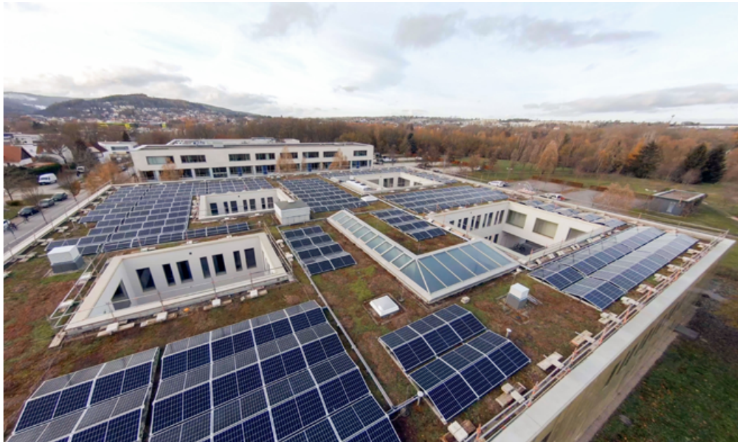
The new photovoltaics system on the institute roof at Fraunhofer IDMT in Ilmenau Photo: Fraunhofer IDMT
