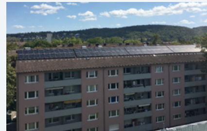
A multi-family building in the Durlach smart district in Karlsruhe. A PV system with a photovoltaic output of 60 kWp was installed on the roof. Photo: Fraunhofer ISE
