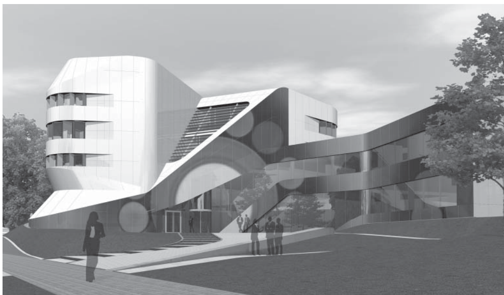
The photomontage shows how the Fraunhofer IAO building in Stuttgart could be fitted with an "efficient design" solar façade. (© Fraunhofer IOF) | Picture in color and printing quality: www.fraunhofer.de/press
