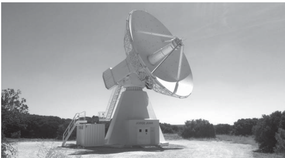
The dish of the radio telescope based in Yebe, Spain, measures more than 13 meters across. Here, the researchers will implement their high-performance radio wave reception technology for the first time. (© Instituto Geográfico Nacional) | Picture in color and printing quality: www.fraunhofer.de/press
