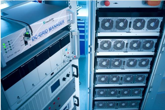
**Picture 2: Electronic power converters and a stationary battery storage system at Fraunhofer IISB.**
