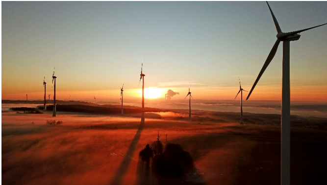
Picture 1: Around 20 percent of electricity in Germany was generated by wind turbines in 2018.
