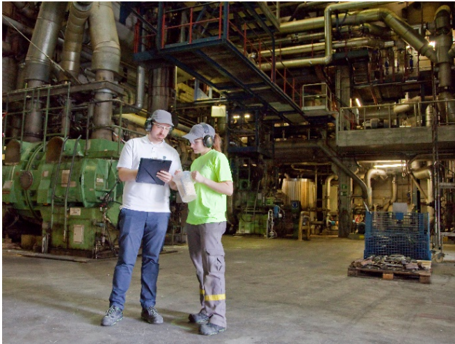
Fig. 1: Many industrial companies, such as those in paper production, use machinery that requires a lot of power. With a production schedule based on generating capacity, such equipment can be operated in an energy-adaptive manner.
