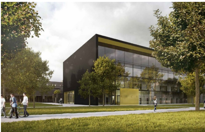
Picture 1: The Fraunhofer Institute for Casting, Composite and Processing Technology IGCV's new facility in Garching was a pilot project designed with digital interior specifications.
