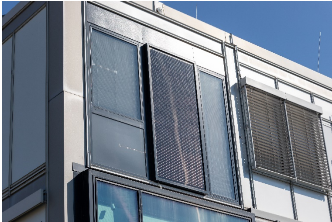
Picture 1 Exterior view of the RE modular facade with a floor-to-ceiling PV element.
