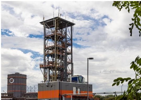
Figure 2: \mu DRAL plant — first direct reduction plant flexibly operated with hydrogen and natural gas in an integrated mill.
