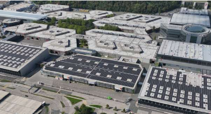
The first photovoltaic systems have been installed on the roofs of the exhibition halls Photo: NürnbergMesse GmbH
