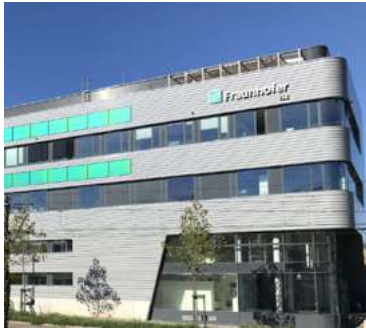
PV modules with a green MorphoColor® structural layer on the wall of the Fraunhofer ISE building Photo: Fraunhofer ISE Benedikt Bläsi
