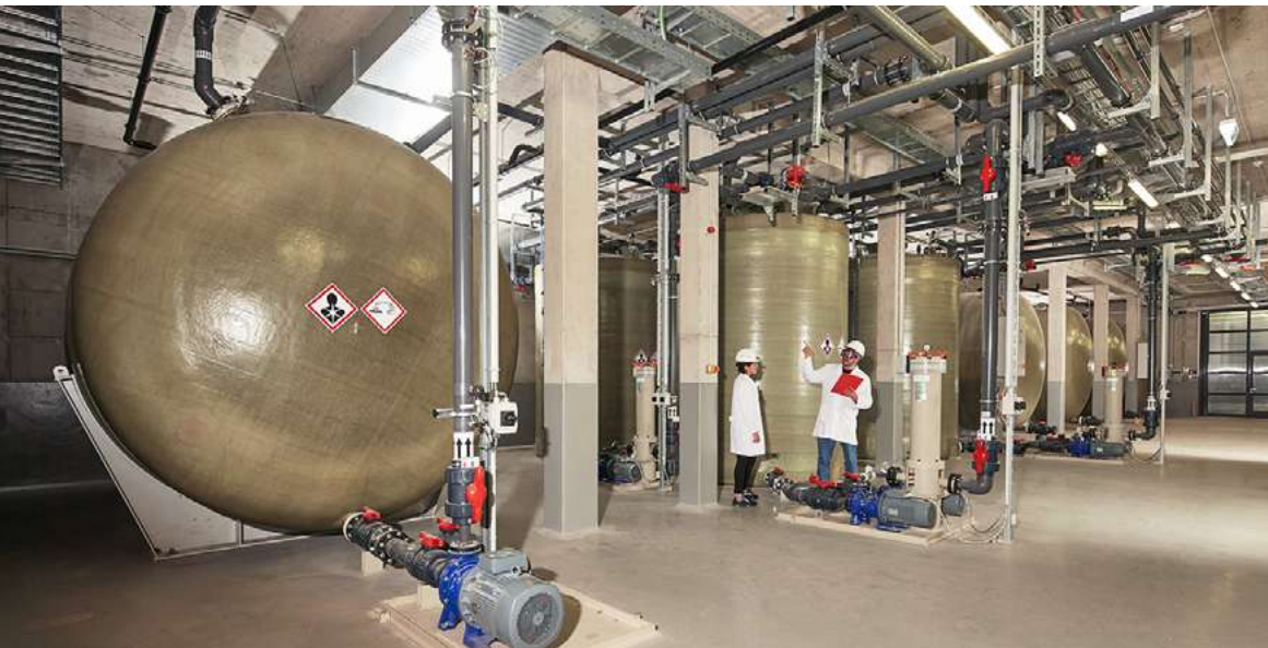
▲ The underground electrolyte tanks for the redox flow battery at Fraunhofer ICT Photo: Fraunhofer ICT
