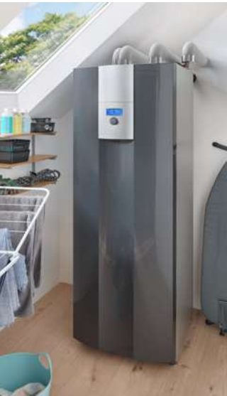
◀ These brine-to-water heat pumps with propane do not require an additional ventilation concept Photo: ait-deutschland
